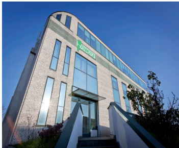
Enerdoor / Finmotor headquarters Milan, Italy
